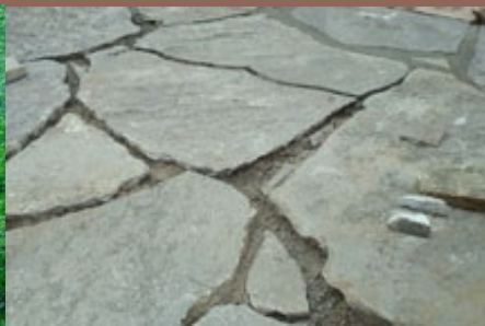
"Repair work in progress"
